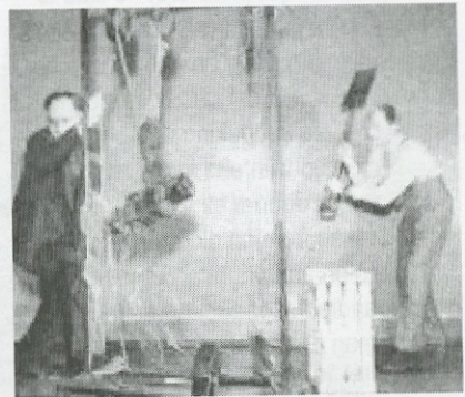
A bomb blast, ship decks splinter, as fire breaks out.
